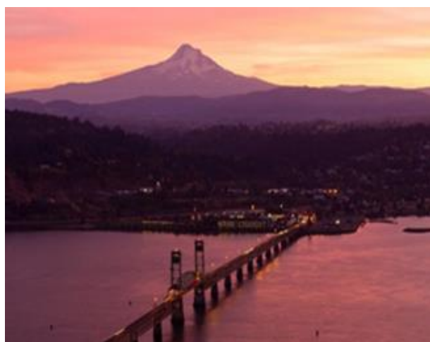
Hood River Bridge on the Columbia River
